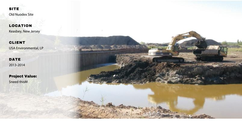
RENOVA self-performed on the construction of a 550-linear-foot sheet pile tieback wall, constructed to allow the prime contractor to safely and effectively excavate radiologically-contaminated soil, while preventing the costly and unnecessary soil disposal caused by sloughing of the excavation walls.
