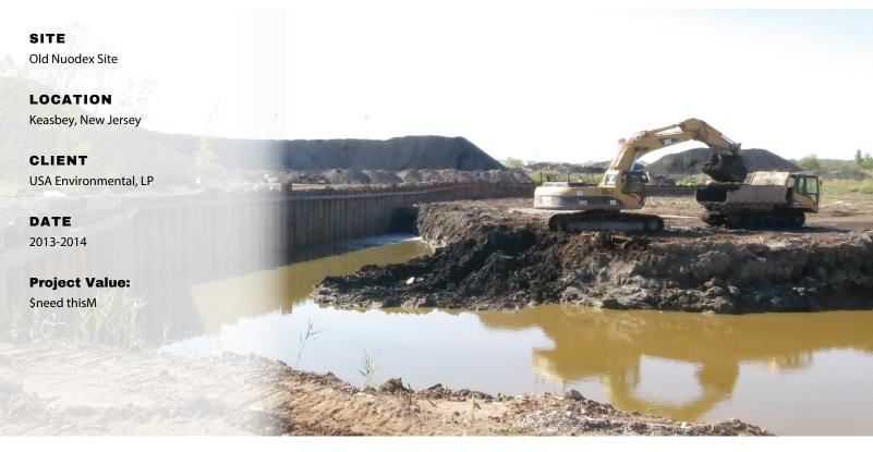
RENOVA self-performed on the construction of a 550-linear-foot sheet pile tieback wall, constructed to allow the prime contractor to safely and effectively excavate radiologically-contaminated soil, while preventing the costly and unnecessary soil disposal caused by sloughing of the excavation walls.
