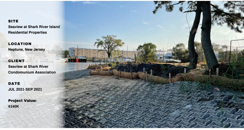
RENOVA was selected as the implementation contractor to stabilize an eroding shoreline utilizing natural and nature-based features (NNBFs) to protect the 200 residential units of a condominium association on Shark River Island in Neptune, New Jersey. RENOVA worked closely with the key stakeholders, with involvement from the engineer of record, American Littoral Society (ALS), New Jersey Department of Environmental Protection and United States Army Corps of Engineers.
