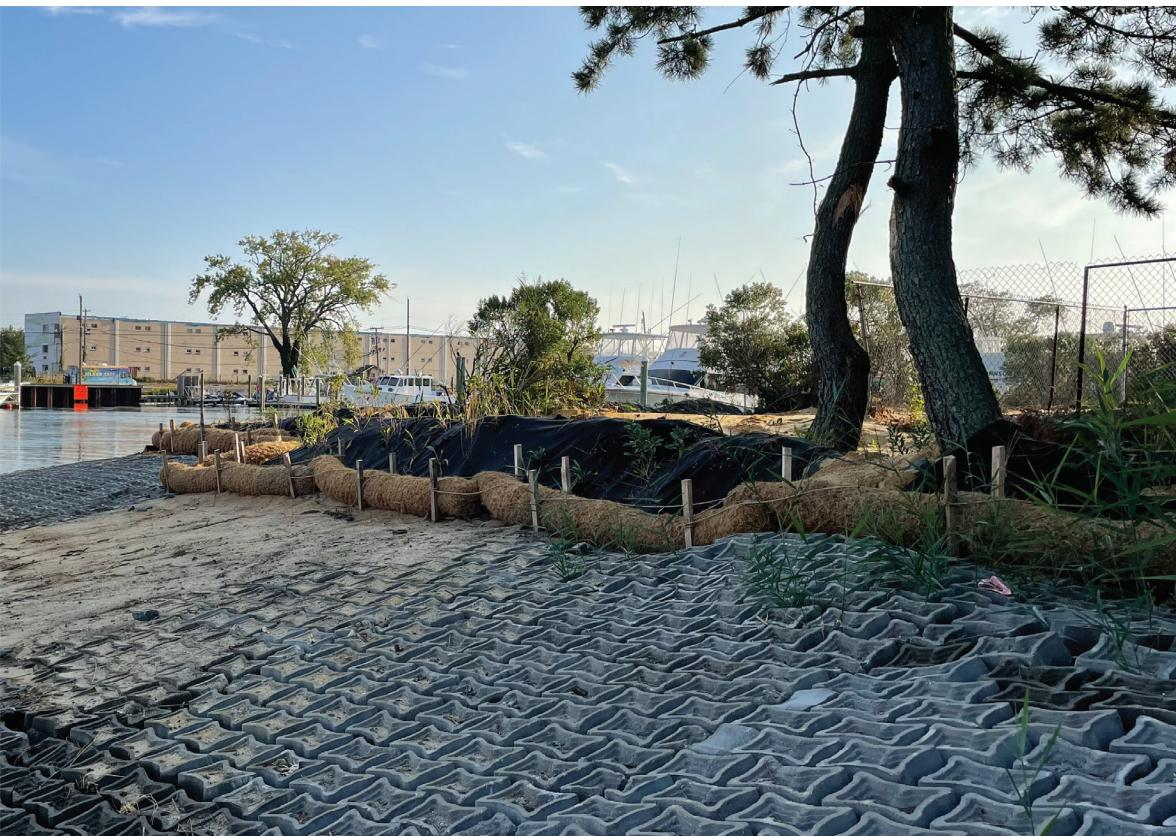
RENOVA was selected as the implementation contractor to stabilize an eroding shoreline utilizing natural and nature-based features (NNBFs) to protect the 200 residential units of a condominium association on Shark River Island in Neptune, New Jersey. RENOVA worked closely with the key stakeholders, with involvement from the engineer of record, American Littoral Society (ALS), New Jersey Department of Environmental Protection and United States Army Corps of Engineers.
